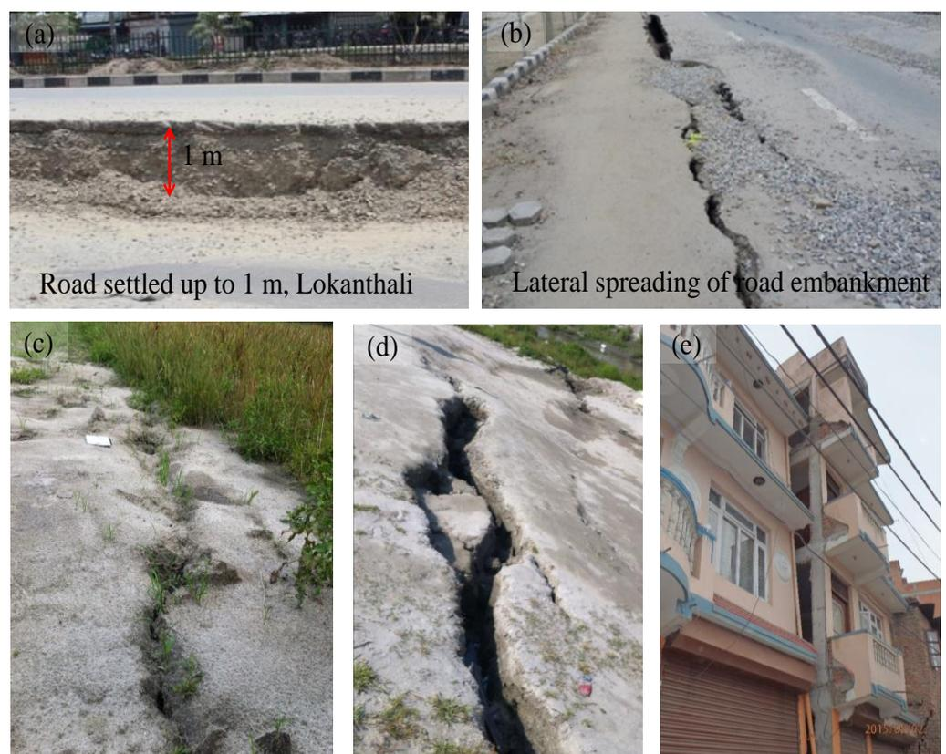
**Figure 2.** Ground liquefaction, settlement, and ground fissures: (a) road settlement at Lokanthali, Bhaktpur; (b) lateral spreading of road embankment, Lalitpur; (c) liquefaction in Bungamati, Lalitpur; (d) liquefaction-induced fissures in Mulpani, and (e) tilted building due to adjacent ground settlement during the 2015 Gorkha, Nepal, earthquake.
